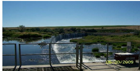
Future winter outfall location at Three Mile Dam.
