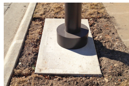
Acceptable Footer Detail
