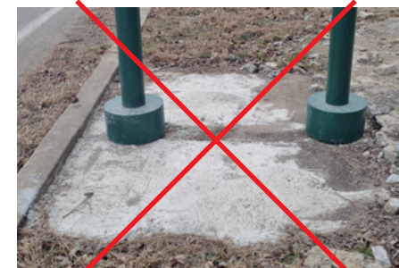
NOT Acceptable Footer Detail
