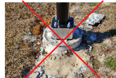
NOT Acceptable Footer Detail
