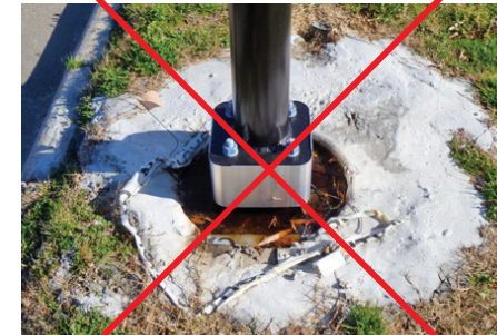
NOT Acceptable Footer Detail
